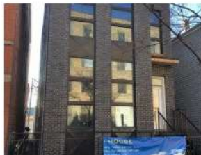
+Plus House, 919 W. Cullerton St., Chicago, IL 60608
